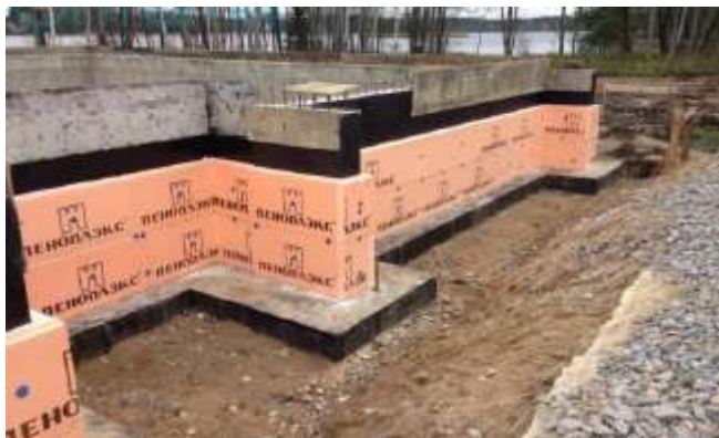
Fig - 4. Thermal insulation and waterproofing of the foundation.
